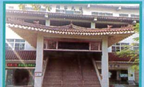
Siaojiuetuei Multifunction Community Center
